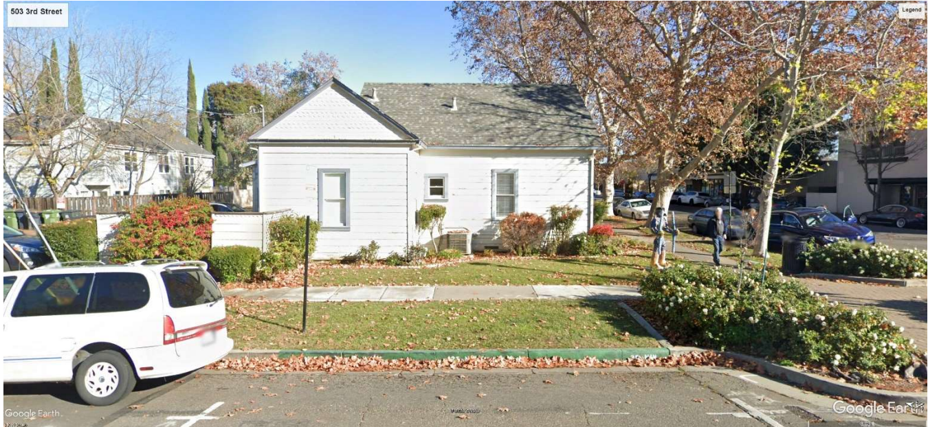
Figure 4 –503 3 rd street, side view (Google Earth 05/30/2023)
